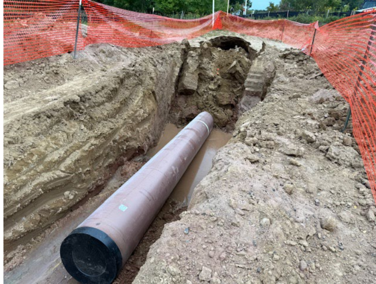
HDD P4-4 completed the pull
