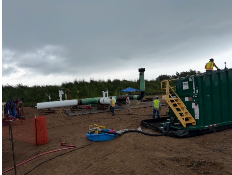
Facing east near MP 0.1, Otis preparing hydrostatic test on fabrication for the Hugo compressor station
