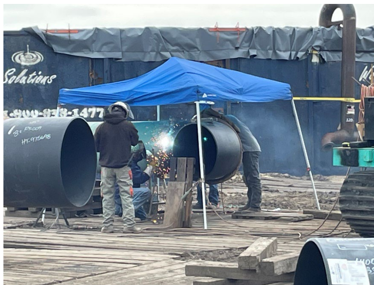
Facing north at MP 34.2, K&K fabricating 36-inch-diameter tie-over piping north of 165th Street
