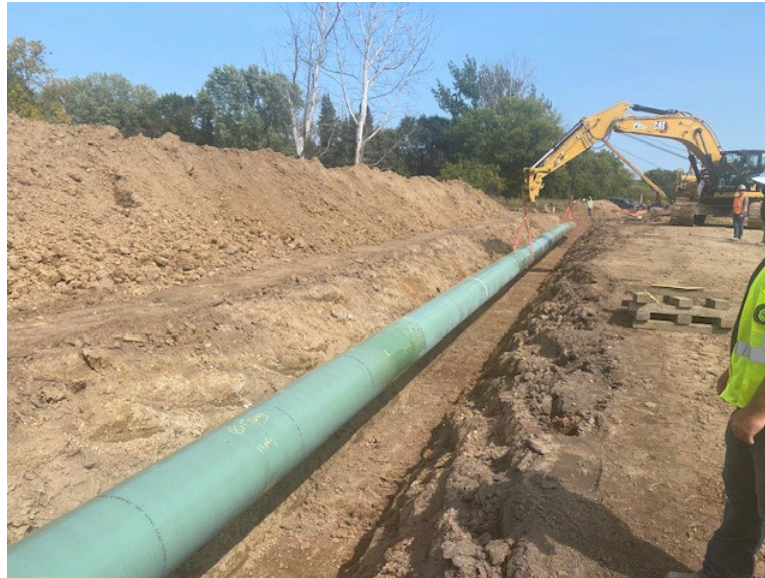
Facing east near MP 1.87, lowering-in ongoing
