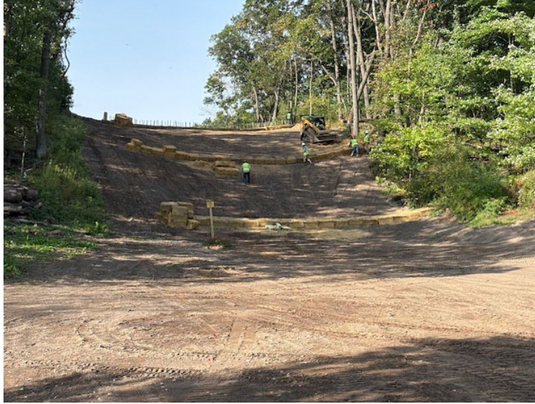
Facing west near MP 2.5, K&K installing slope breakers
