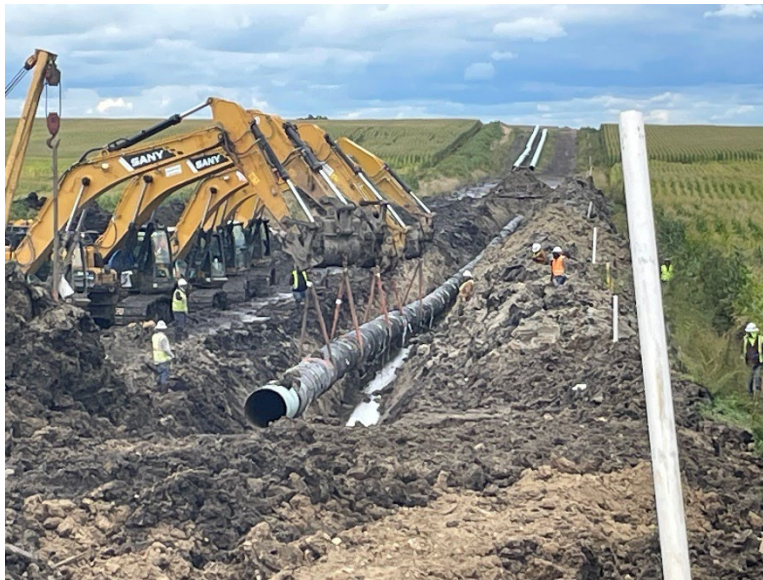
Facing north at MP 32.38, K&K lowering-in mainline pipe north of 140th Street
