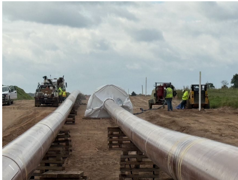
Facing south near MP 1.15, Otis sandblasting bore pipe for HDD P4-2
