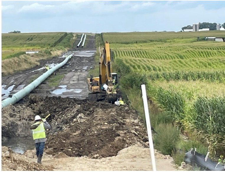
Facing north at MP 32.4, K&K removing topsoil from over D-line north of 140th Street
