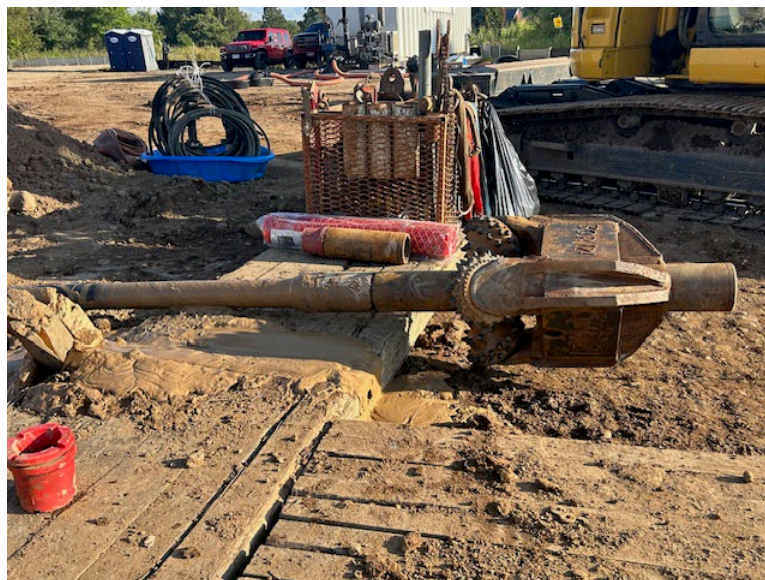
HDD P4-1 commenced the ream pass
