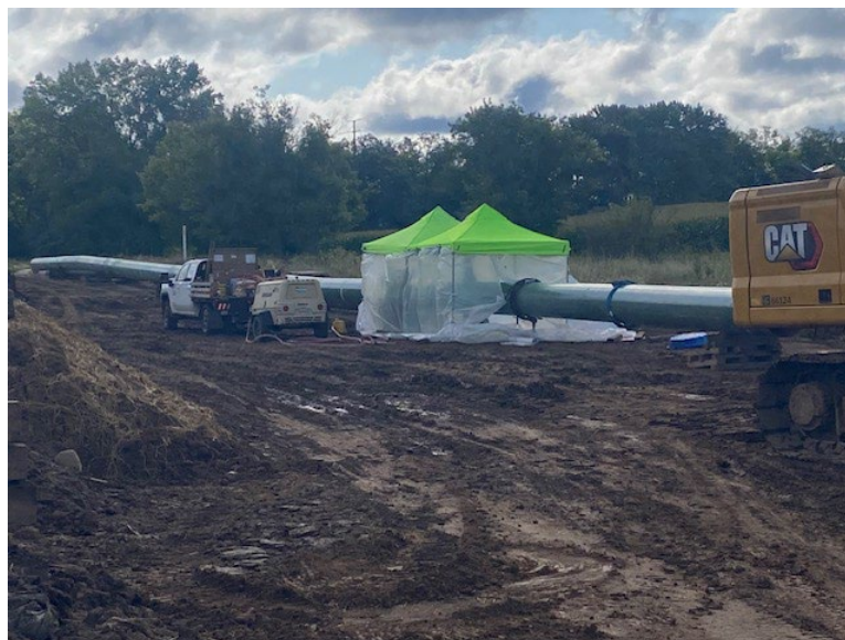
Facing south, near MP 1.8, sandblasting and coating ongoing
