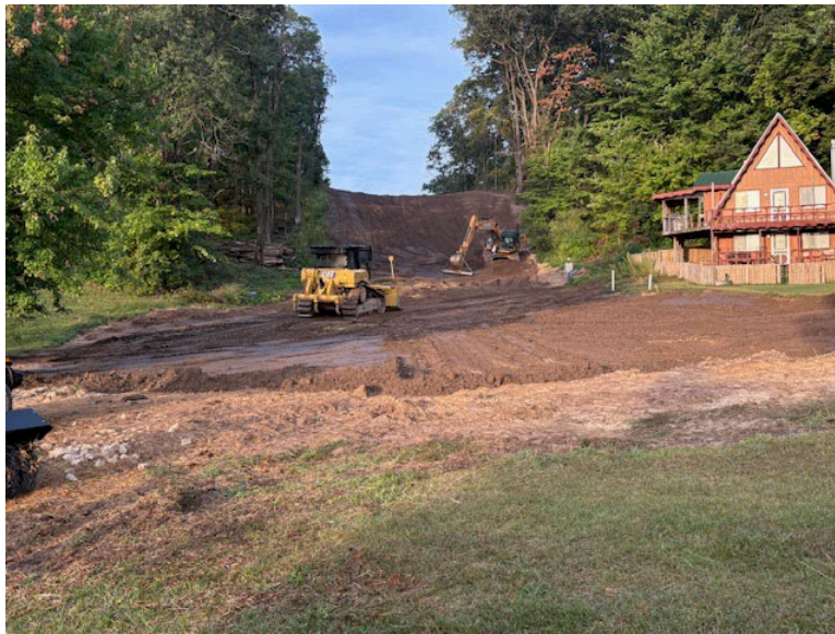
Facing west near MP 2.5, K&K restoring topsoil
