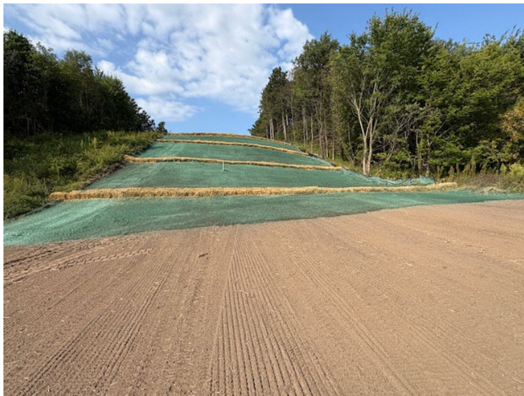
Facing west near MP 3.2, hydroseeding completed
