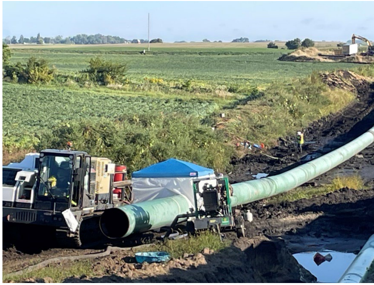
Facing northwest at MP 31.6, K&K sandblasting and coating north of County Road 9/135th Street
